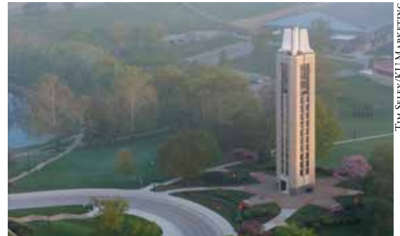
The Campanile and the base environs before renewal
