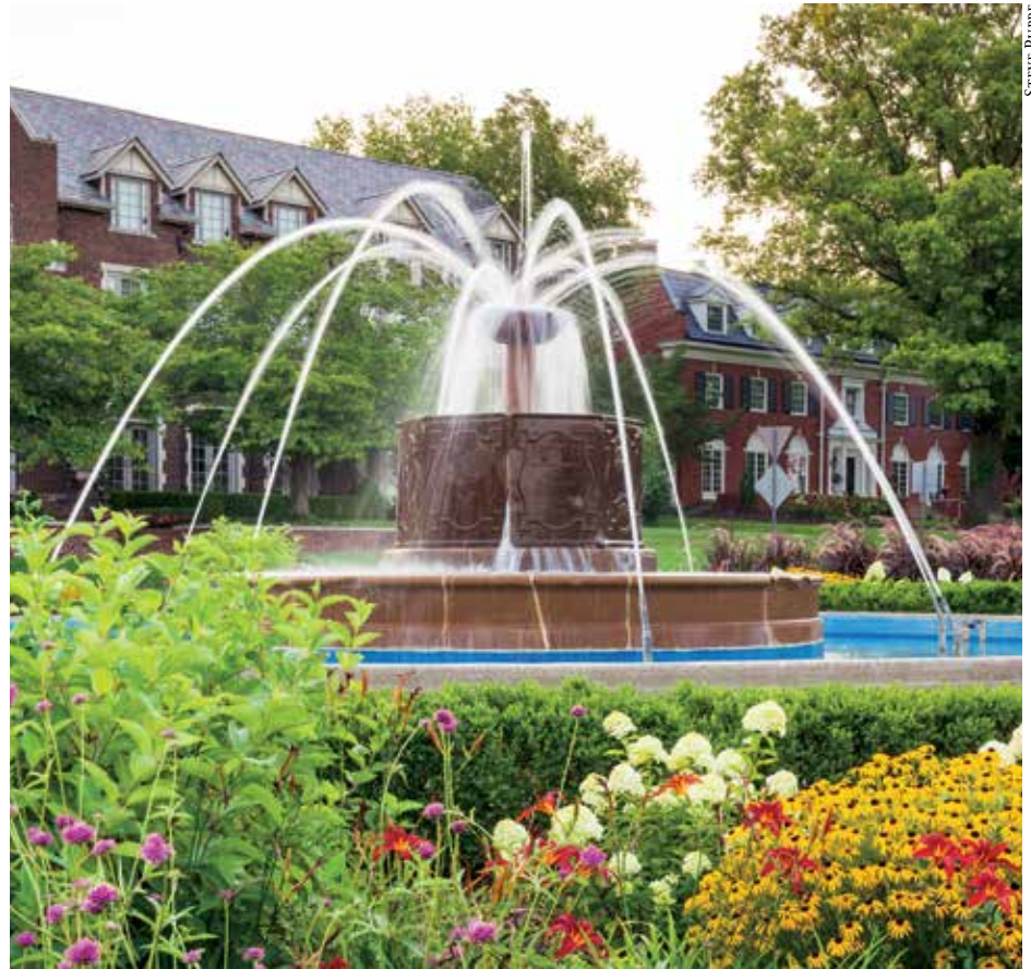
Chi Omega Fountain, shortly before its center structure was removed. Note the water pouring from joints in octagonal metal basket.
