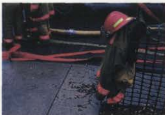
On the cover: Lightning struck Hoch Auditorium June 15, igniting a fire that gutted the structure and caused $13 million damage—the most costly fire in modern Lawrence history.
