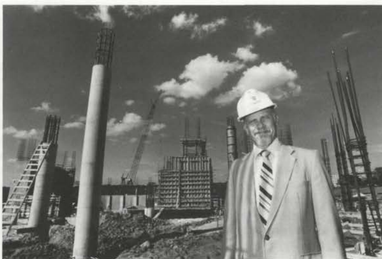
CONCRETE PROGRESS: Wiechert surveys the upcoming Lied Center, to open in 1993.
