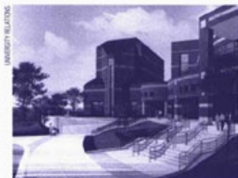
SITE FOR SOUND: Construction begins this fall on the Bales Organ Recital Hall to adjoin the Lied Center.
