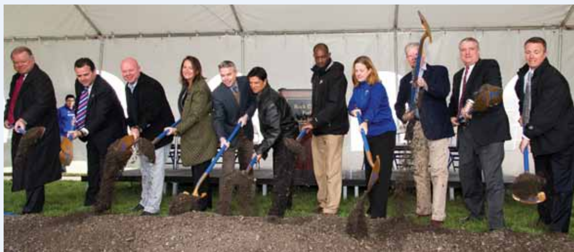
Diamond Dixon (p. 32), Dale Seufferling (above, l-r), Sheahon Zenger and Thomas Fritzel dug in to help launch what Zenger says is Kansas Athletics' largest building project since the construction of Memorial Stadium and Allen Field House.
